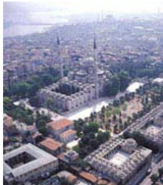
Figure 4. Arial View of the Fatih Mosque Complex and Sahn-i Semân Madrasas
